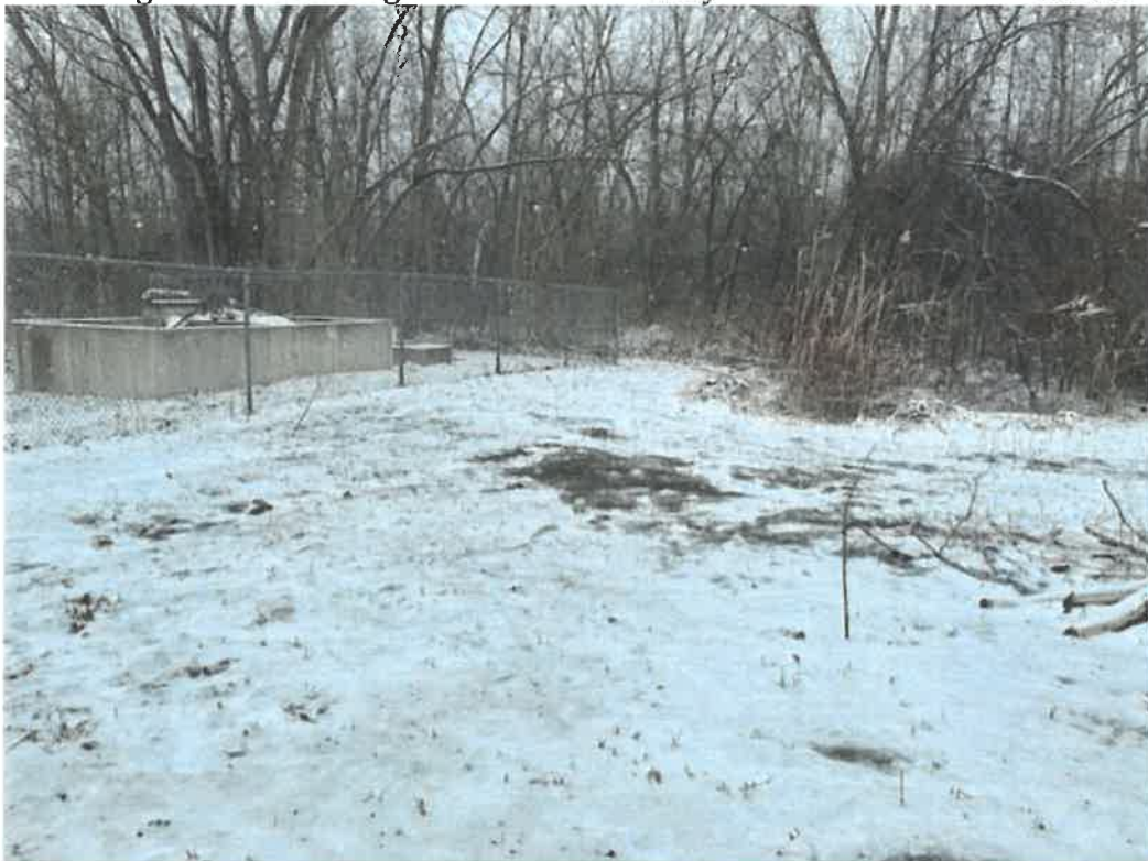
Ponding behind buildings next to WWTP. May be effluent based on odors.
