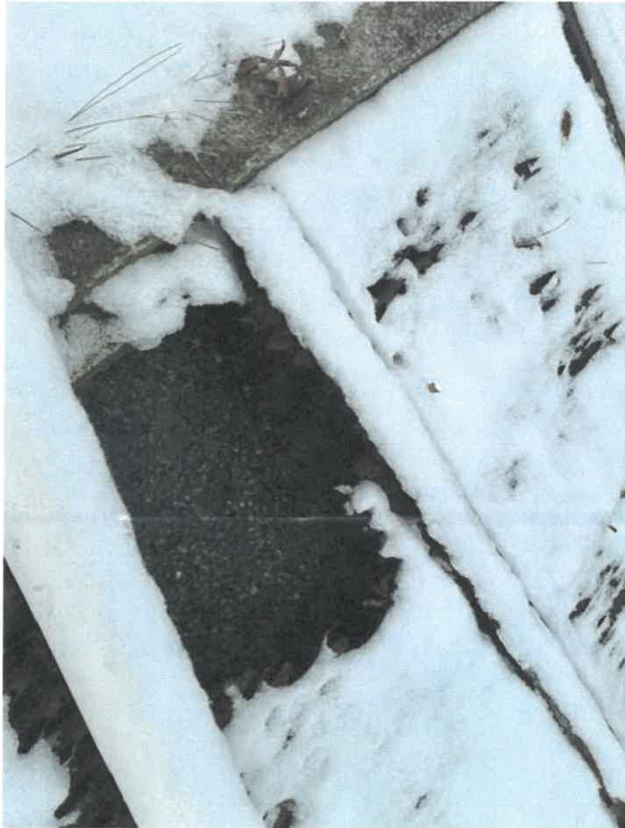
Overly full aeration tank and broken grate.
