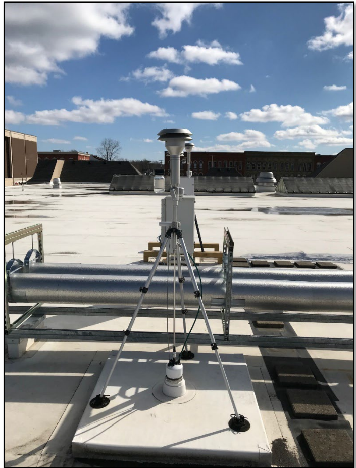
PM 2.5 Monitor Intake - JFS building in Painesville.
