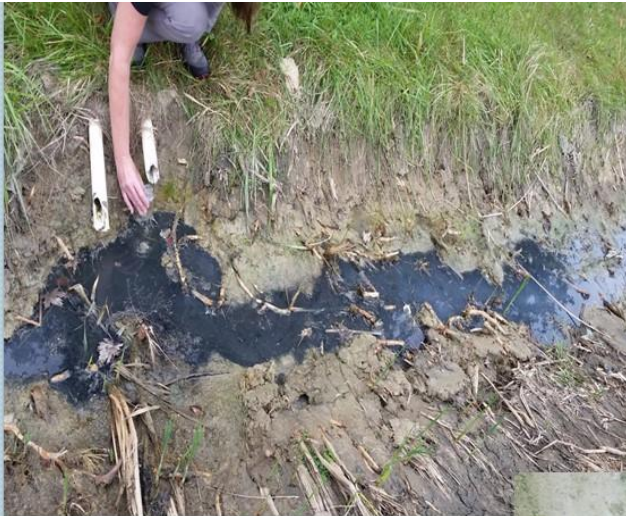
Sewage from failing septic systems
