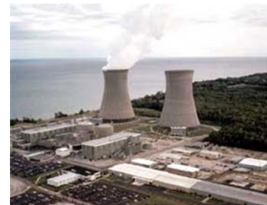
Perry Nuclear Power Plant, Aerial View
